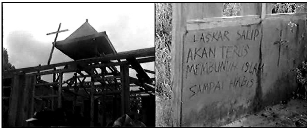
Figure 6.4 Examples of the pictures of burnt mosques and graffiti on the walls that insult Islam
